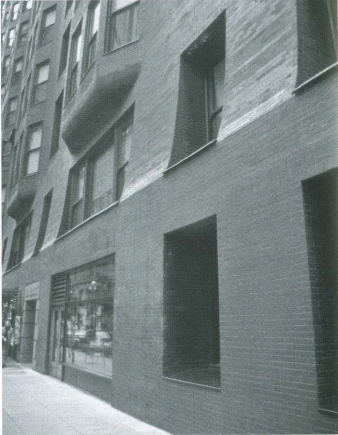
Figure 2 Thickening of the walls on the lower levels Merwood-Salisbury, Chicago 1890: The Skyscraper and the Modern City, 2009
